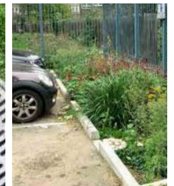
Figure EA.10. Intervals to allow water into rain garden
